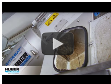
Video: Mechanical preliminary wastewater treatment - example: municipal WWTP Weiden https://www.youtube.com/watch?v=vyieOQUR_9o
