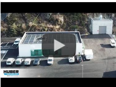
Video: Complete wastewater treatment at the Øygarden WWTP in Norway https://www.youtube.com/watch?v=KU2awn3DP68
