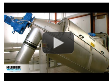
Video: HUBER Screw Thickener S-DRUM - here at a municipal WWTP https://www.youtube.com/watch?
