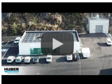
Video: Complete wastewater treatment at the Øygarden WWTP in Norway
