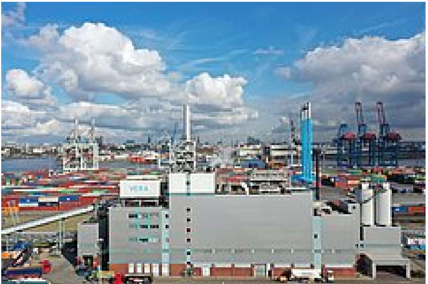
The VERA II plant is located in the port of Hamburg. (© HAMBURG WASSER)
