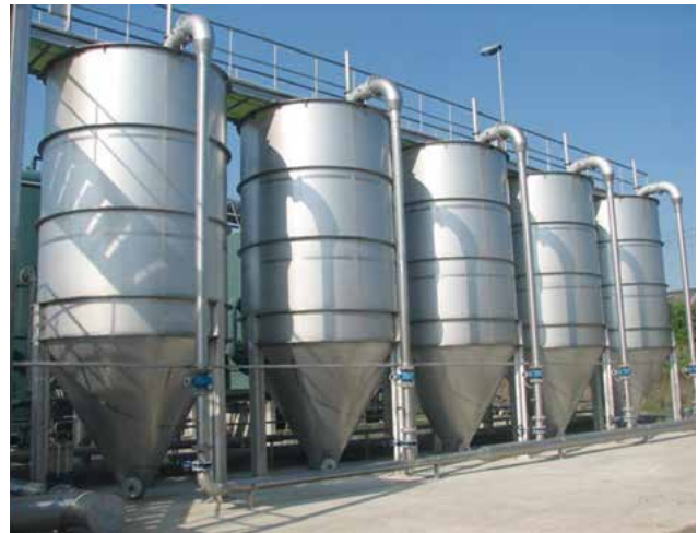
HUBER Sandfilter CONTIFLOW® 72, Montebello, Italy.
