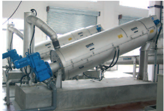
ROTAMAT® RoS 3 screw presses in Kuching, Malaysia
