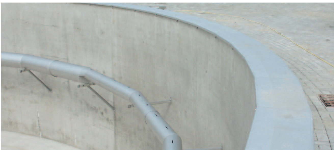
The covering protects the scraper trackway.
