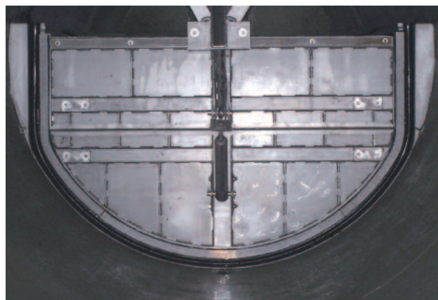
Closed flushing gate for a circular profile DN 2000
