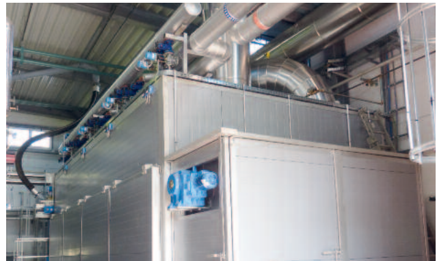
HUBER Belt Dryer BT for sewage sludge drying up to > 90 % DS
