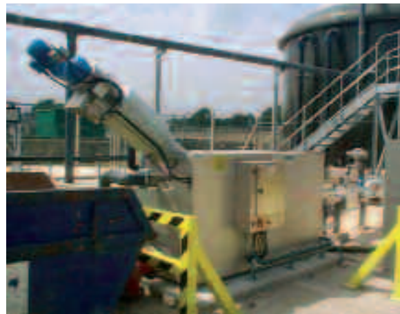
Outdoor installation of a ROTAMAT® Sludge Screening Plant
