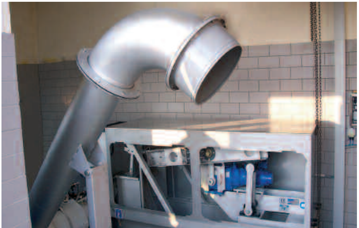
Compact curved bar screen CurveMax® for reliable separation of solids from wastewater
