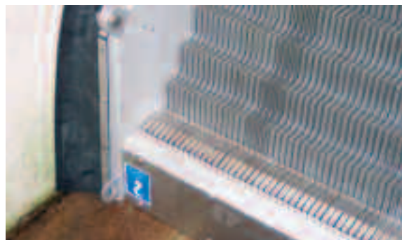
STEP SCREEN® installed in the customer's channel
