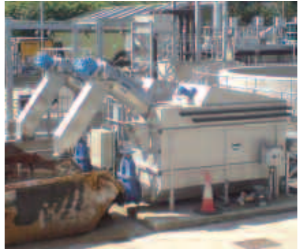
ROTAMAT® Membrane Screen size 1400 with 1 mm mesh size
