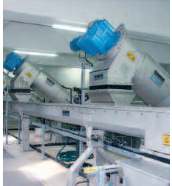
RoMem Screen with a fine mesh for removal of hairs and fibres prior to a hollow fibre membrane plant
