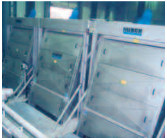
STEP SCREEN® Vertical SSV with a steep installation angle (70°/75°) for deep channels
